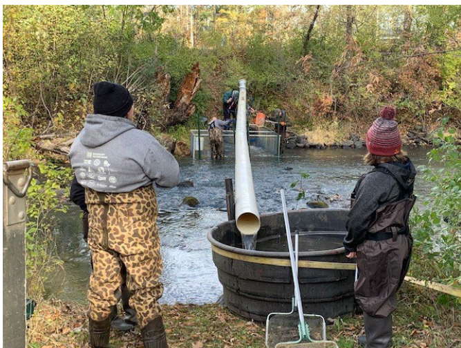
Fingerling muskies are netted as they come out of a rearing pond. From there they get a ride across the Grindstone River on the "fish flume" into a holding tank.
